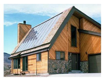
Caption: This home in Colorado uses solar energy to heat water for use inside the home. The black solar collectors on the roof capture and concentrate solar energy to heat water. Source: http://www.howstuffworks.com/environmental/green-tech/sustainable/solar-water-heater.htm
